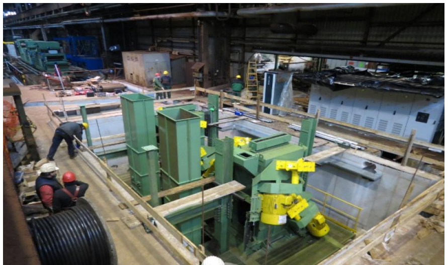
Photos: 3D picture shows a 15m high Siapro machine for coil steel strips mechanical cleaning. Photo during assembly at final location.
